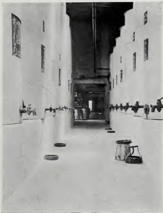
FIG. 54.—Varnish Storage. Louisville Varnish Co.
